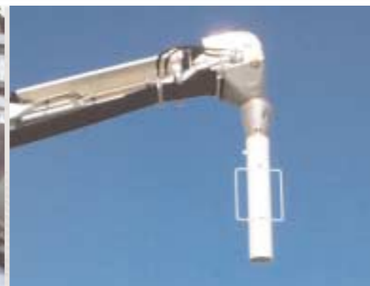
Cardanic conveyor for the easy distribution of concrete
